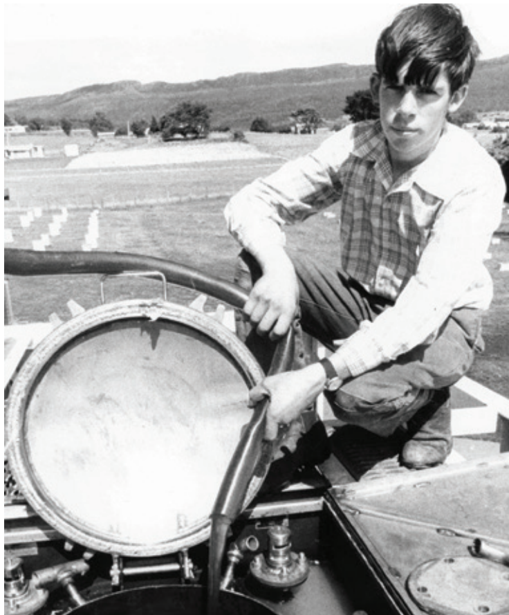
Filling a bulk container for the UK by pump line
